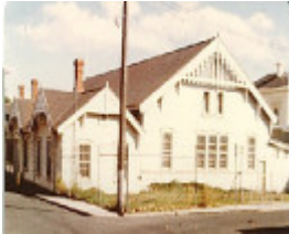
B5133 Drill Hall
