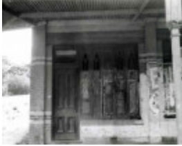
B2204 Langslow's Building Front
