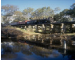
B6981 Muckleford Creek bridge
