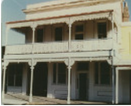
B5265 Former Albion Hotel
