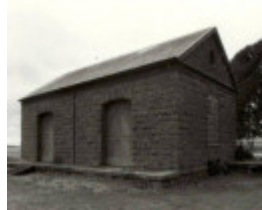
B3931 Bluestone Goods Shed
