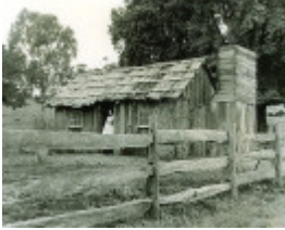
B2835 Re-erected Hut & Cemetery, NARINGAL
