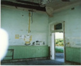
B5431 Railway Station, Koroit pre restoration
