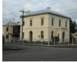
Former Bank of Victoria/ Moyne Shire Office
