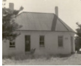
B0764 Former Merrijig Hotel
