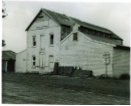
B0765 Warehouse/Butter Factory
