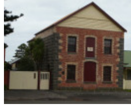
B0765 Warehouse/ Butter Factory
