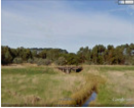
B7057 Burchett Creek Bridge (Google Earth image)
