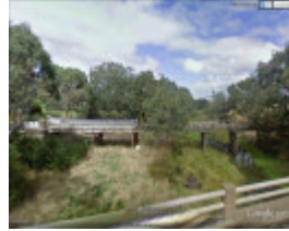
B6521 GoogleEarth Image Ellerslie Bridge
