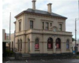
B0862 Post Office (former) Port Fairy
