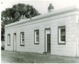
B2862 Seacombe House Sackville Street, Port Fairy
