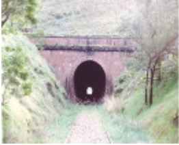
B5486 Cheviot Railway Tunnel
