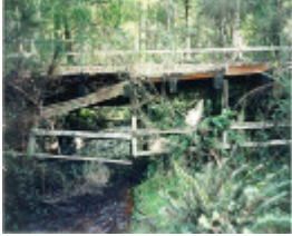
B6439 Wilks Creek Bridge
