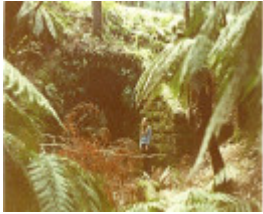
B5804 Big Culvert
