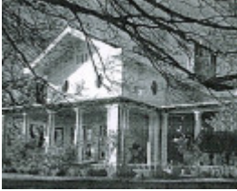
B1456 Alanvale Homestead, Campbells Bridge
