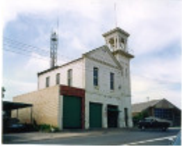
B6354 Stawell Fire Station
