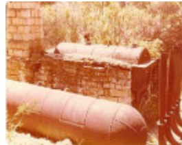
B4361 power plant, Heatherlie Quarry, Ledcourt
