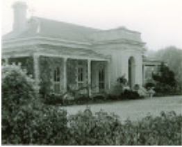
B2845 Kirkella Homestead, Campbells Bridge
