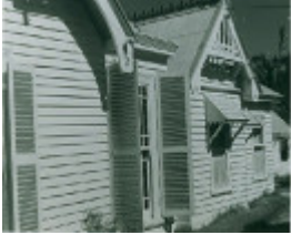
B3570 Navarre Station
