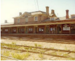
B5134 Stawell Railway Station
