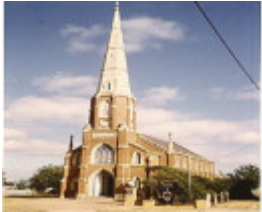
"B1699 St Matthews Uniting Church, Stawell"
