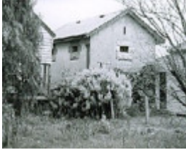
B1395 Stawell Lockup, Stawell
