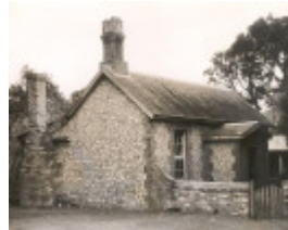
B0657 Swan Water South Kitchen
