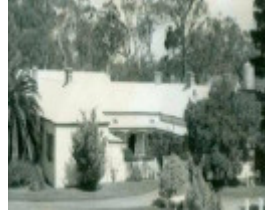
B1319 Tottington Homestead Courtyard
