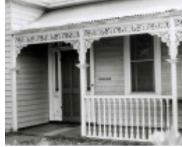
B2180 Warraine Front Verandah
