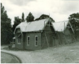
B4925 Former Post Office
