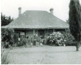
B1837 Chock & Log Cottage, Poowong
