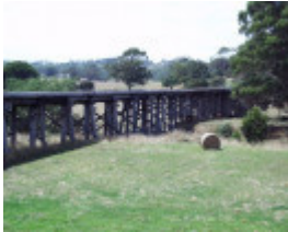
B6952 Tarwin River East Branch Railway Bridge
