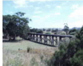
B6952 Tarwin River East Branch Railway Bridge
