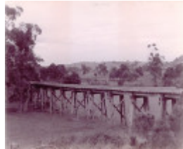
B6952 Tarwin River East Branch Railway Bridge
