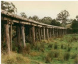
B6953 Koonwarra Rail Bridge
