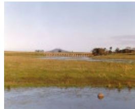
B6909 Railway Bridge
