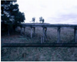
B6909 Railway Bridge
