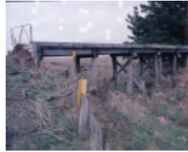
B6909 Railway Bridge
