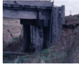
B6909 Railway Bridge
