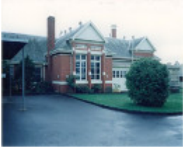
B6399 Hamilton Base Hospital Complex
