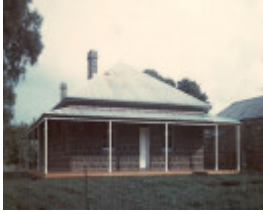
B3698 Lyne Homestead & Out Buildings
