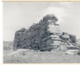
B1224 Old Chimney
