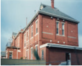
B5027 Administration Building
