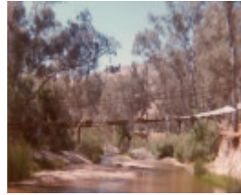
B5279 Suspension Bridge
