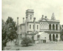
B1357 Noorilim Homestead South West View
