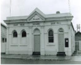
B1167 Former Shire Hall 344 High St Nagambie
