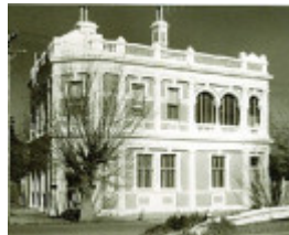
B5170 Former Colonial Bank
