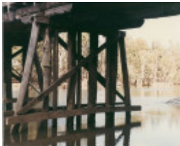
B6849 Mitchellstown Bridge piers
