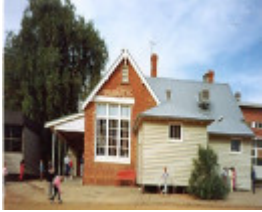
B5642 Former Primary School No 1142
