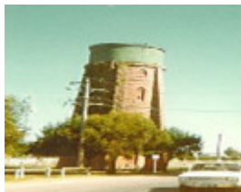
B4866 Water Tower, Monash Drive
