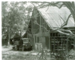
B4559 Stable Building Noorongong
