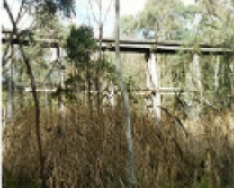
b6951 Darbyshire Creek No 2 Bridge
