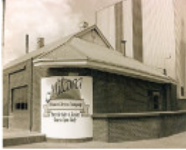
B6274 Milawa Cooperative Dairy Co Ltd
