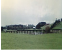
B6911 Rail Bridge Dennington
