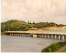
B6701 Hopkins River Timber Truss Bridge
