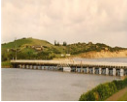
B6701 Hopkins River Timber Truss Bridge
