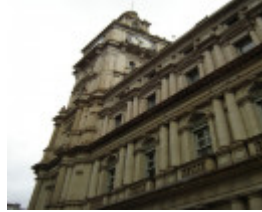
h00903 gpo bourke street2
